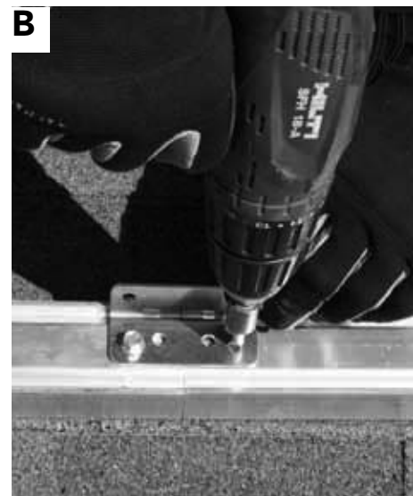
B A drill driver may be used to install the four (4) self-drilling screws. Over-tightening the screws will result in stripped threads.
