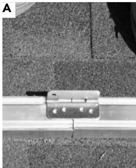
A Retainer/splice may be installed on the top or bottom flange of the beam. At least 1 retainer must be placed over an attachment for each run of beams
